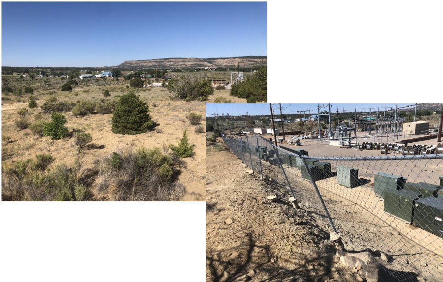
Future sight of the Cuba Solar Array project and a need for the redesign and expansion of the JMEC operations yard due to erosion.
